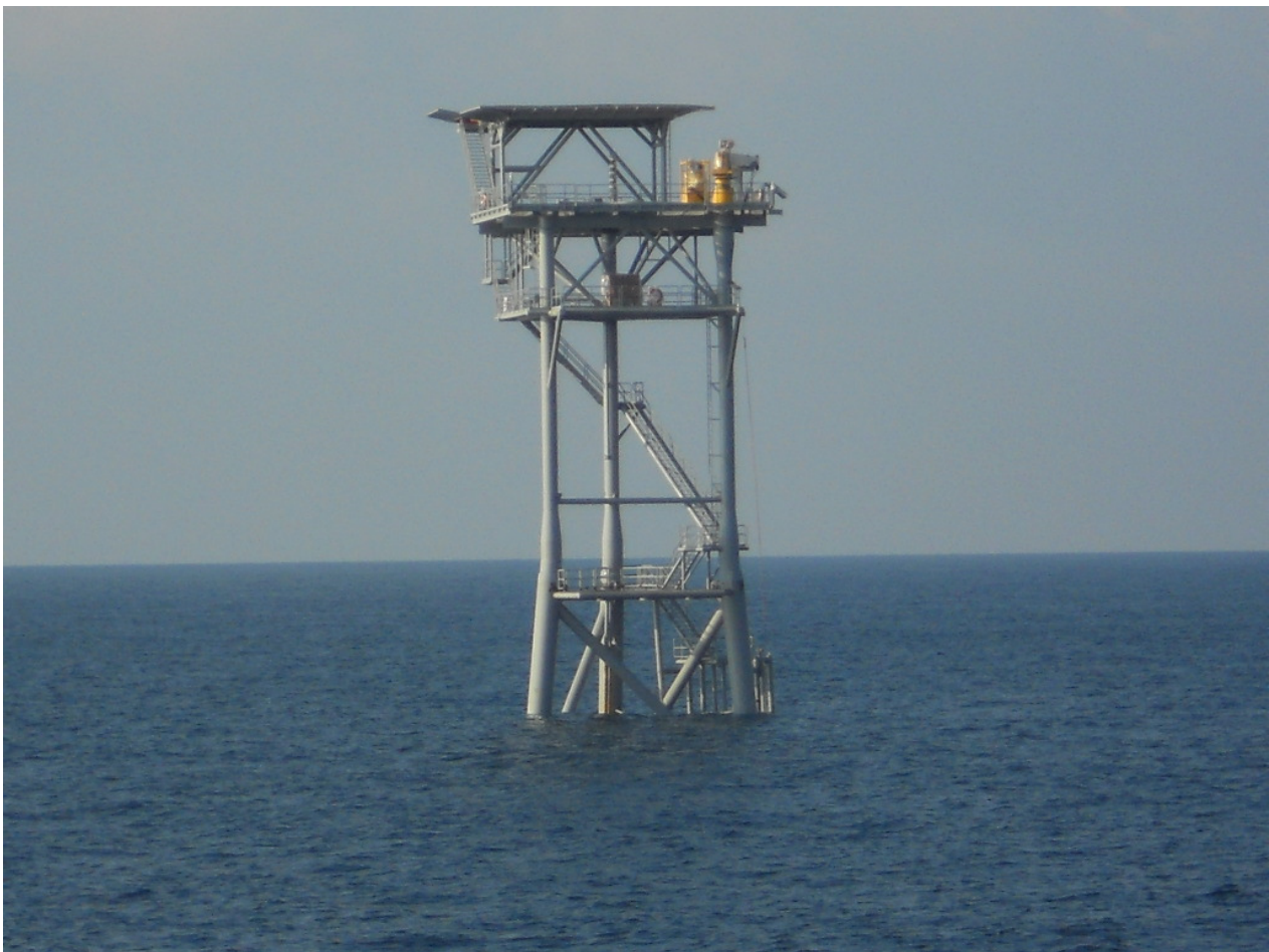
Photo of the completed GA A133 platform
