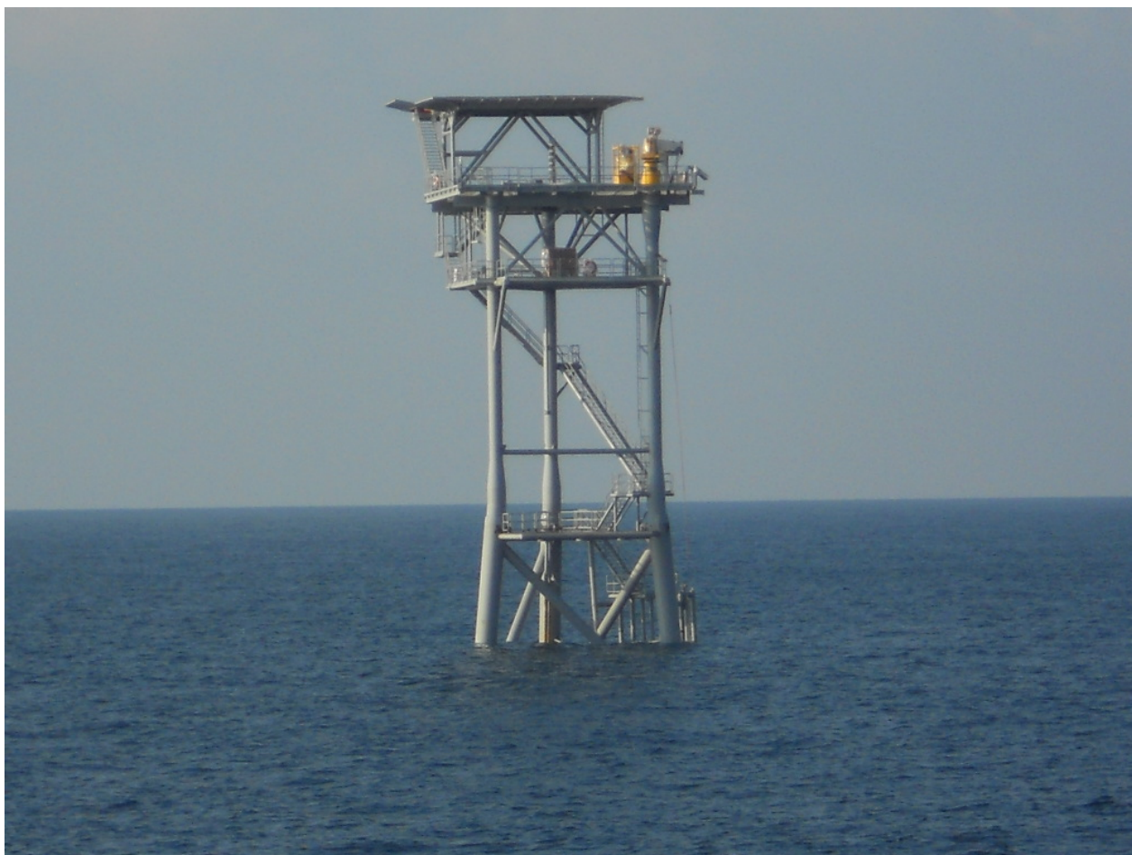
Figure 6: Photo of the completed GA A133 platform
