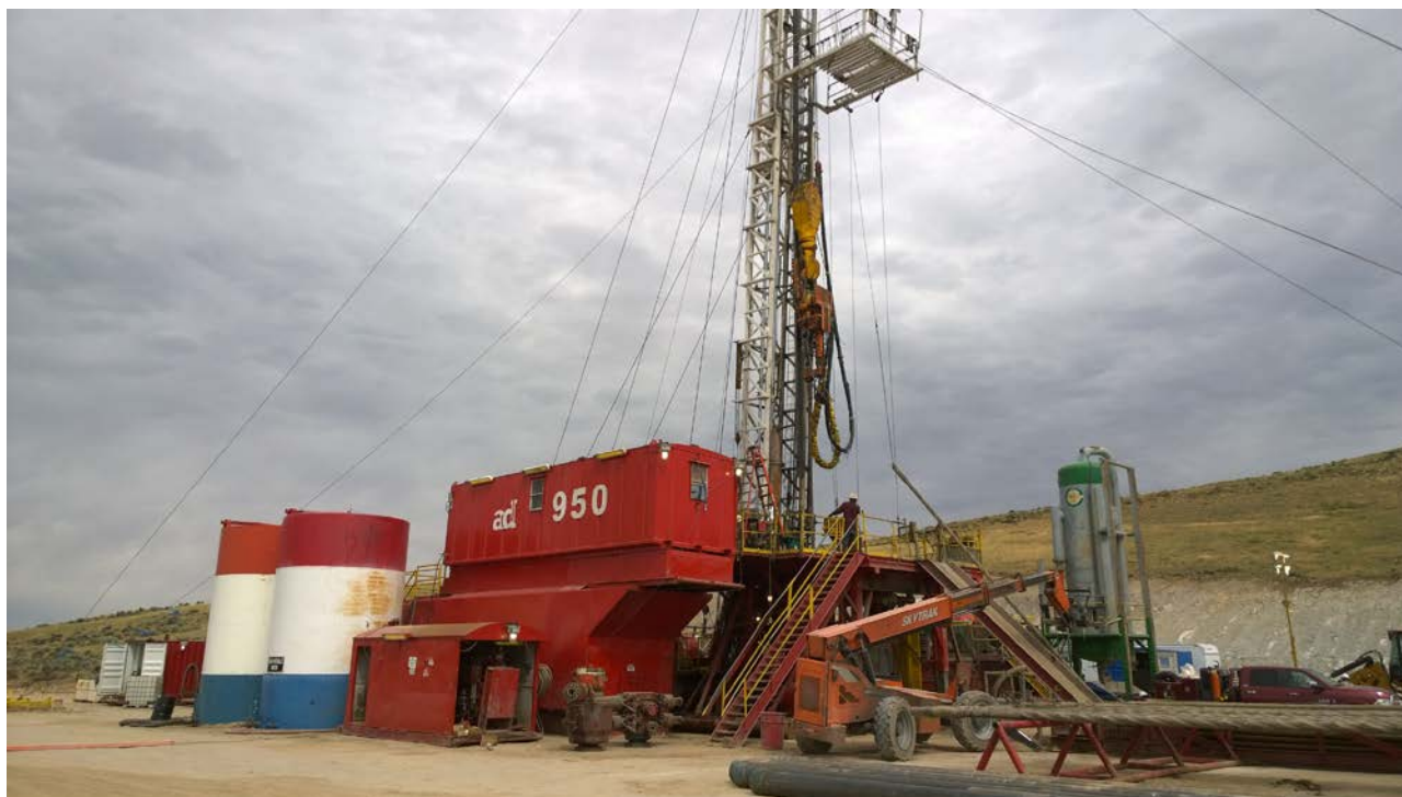
Drilling Rig on McKee 5-16 Well Location
